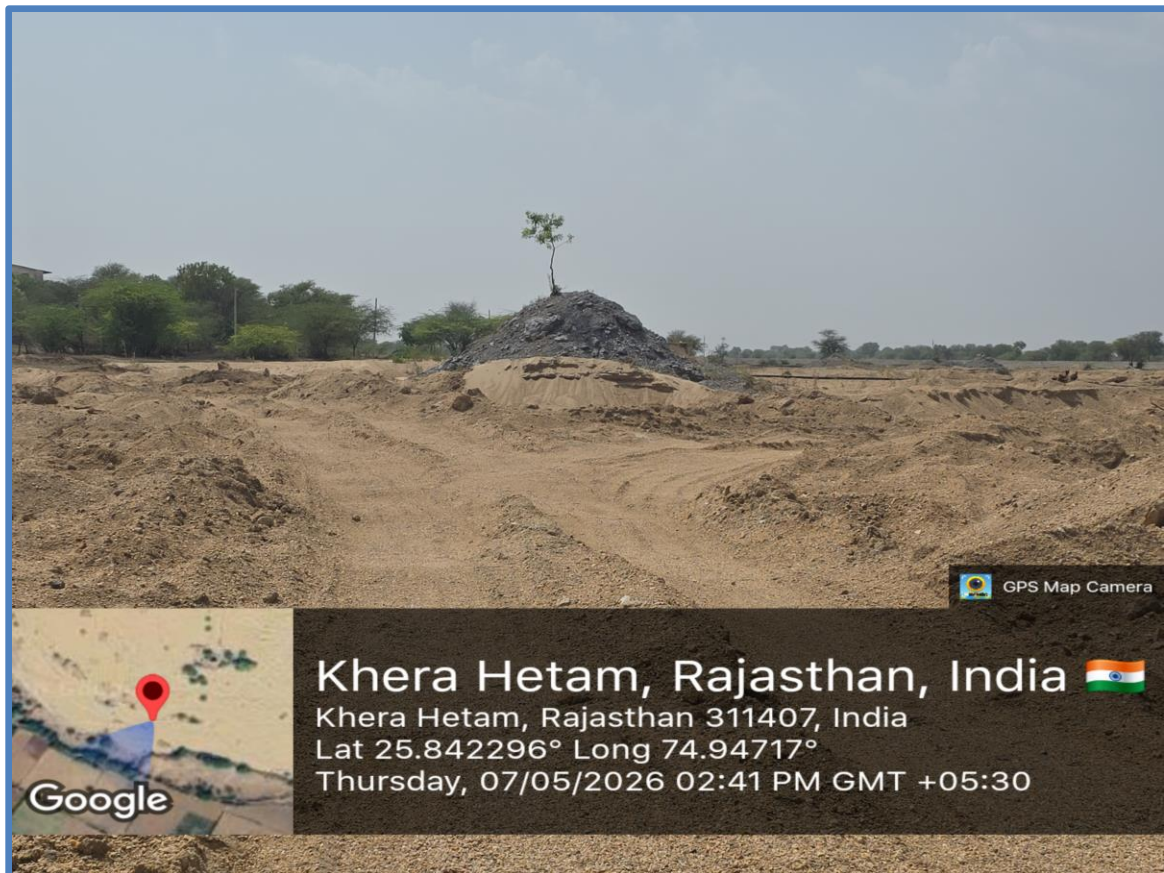
Figure 15 : Khari Riverbed Mining Area (Towards Khera Hetam), depicting sign of mining done and the open well 03.
