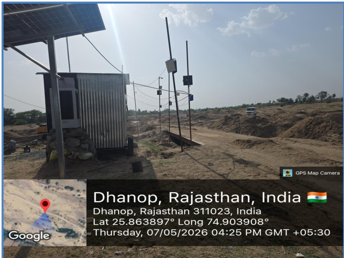
Figure 24: Weighbridge & CCTV Camera Surveillance & Solar plate structure at Khari Riverbed Mining area, Dhanop Mining Point 2
