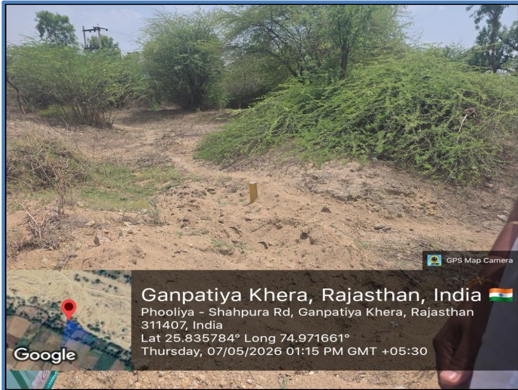
Figure 7: Boundary demarcation pillar observed at the lease area. The Joint Committee verified the presence of pillars but instructed the lessee to raise their heights for better visibility as per statutory guidelines.
