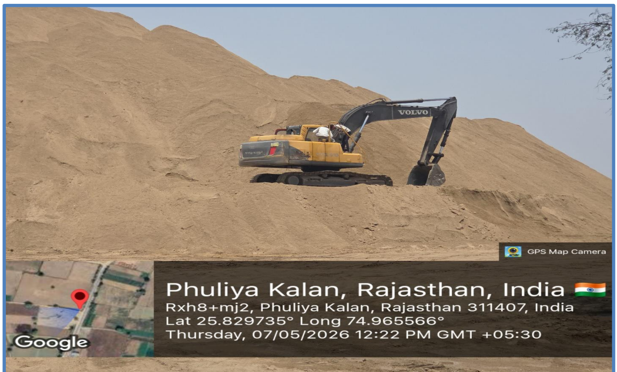
Figure 2: River Sand Stock Handling at Transit Point 01
