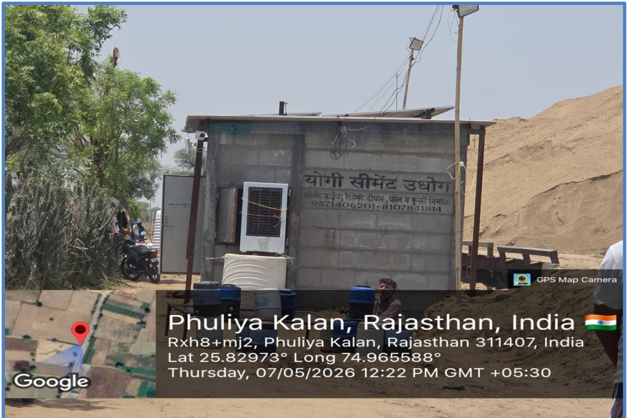
Figure 3: Weighbridge and CCTV installed at Transit Point 01, Phuliya Kalan
